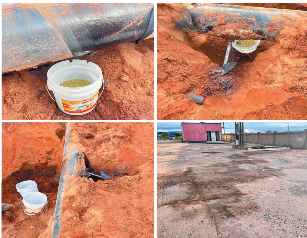
Figure 31: TAZAMA pipeline that was pierced and connected to a one-inch pipe linked to a petroleum storage underground tank of the nearby petroleum retail outlet
